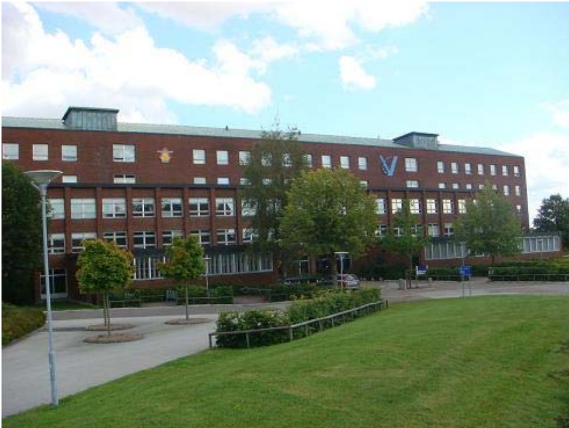
(Picture: Lund University Engineering Department V-huset)
