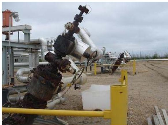
SAGD method (Left : Pattern diagram of SAGD method Right : Deviated well head)
